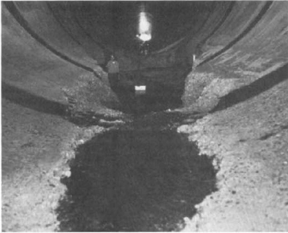
Figure 1.1: Cavitation damage in the spillway tunnel of the Yellowtail Dam, Montana (Arndt, 1981). Courtesy of the US Bureau of Reclamations.
