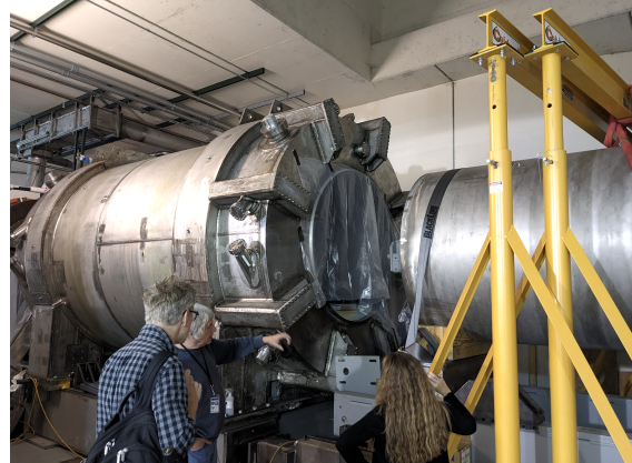
(b) The Heat and Radiation Shield being inserted inside the Production Solenoid (in October 2025)
