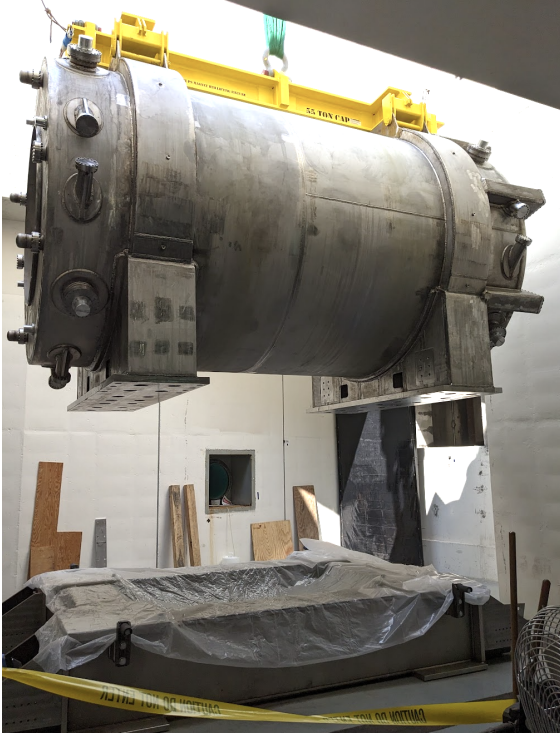
(a) The Production Solenoid being lowered in its final location (in August 2025)
