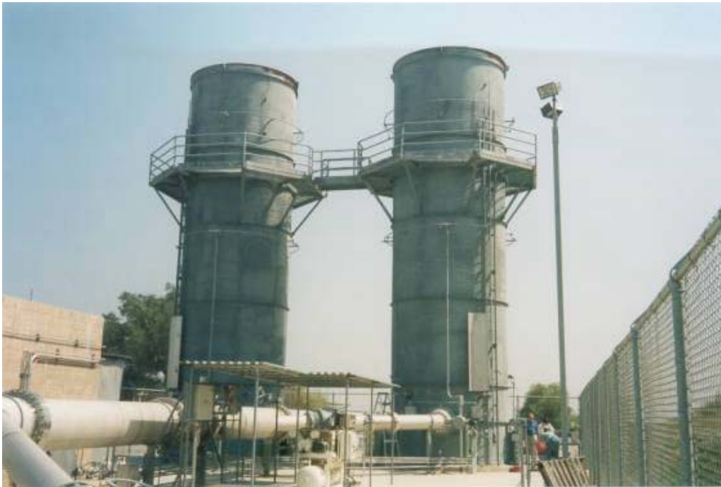
Figure 3-1: Landfill flare station.
